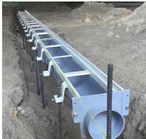
Rebar attachments prevent floating
